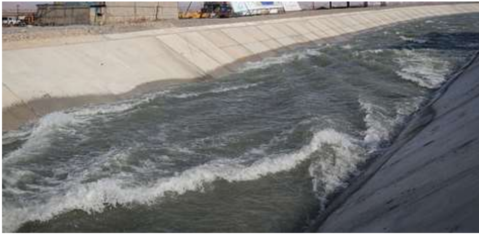
Figure 5. A view of the water transfer channel of the Kani Siu project. 70 km transmission line with an annual capacity of 300 million water from the Badinawe Dam to the Gadar River. Source: www.president.ir
